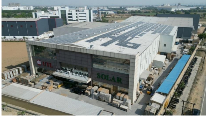
Greater Noida Facility
